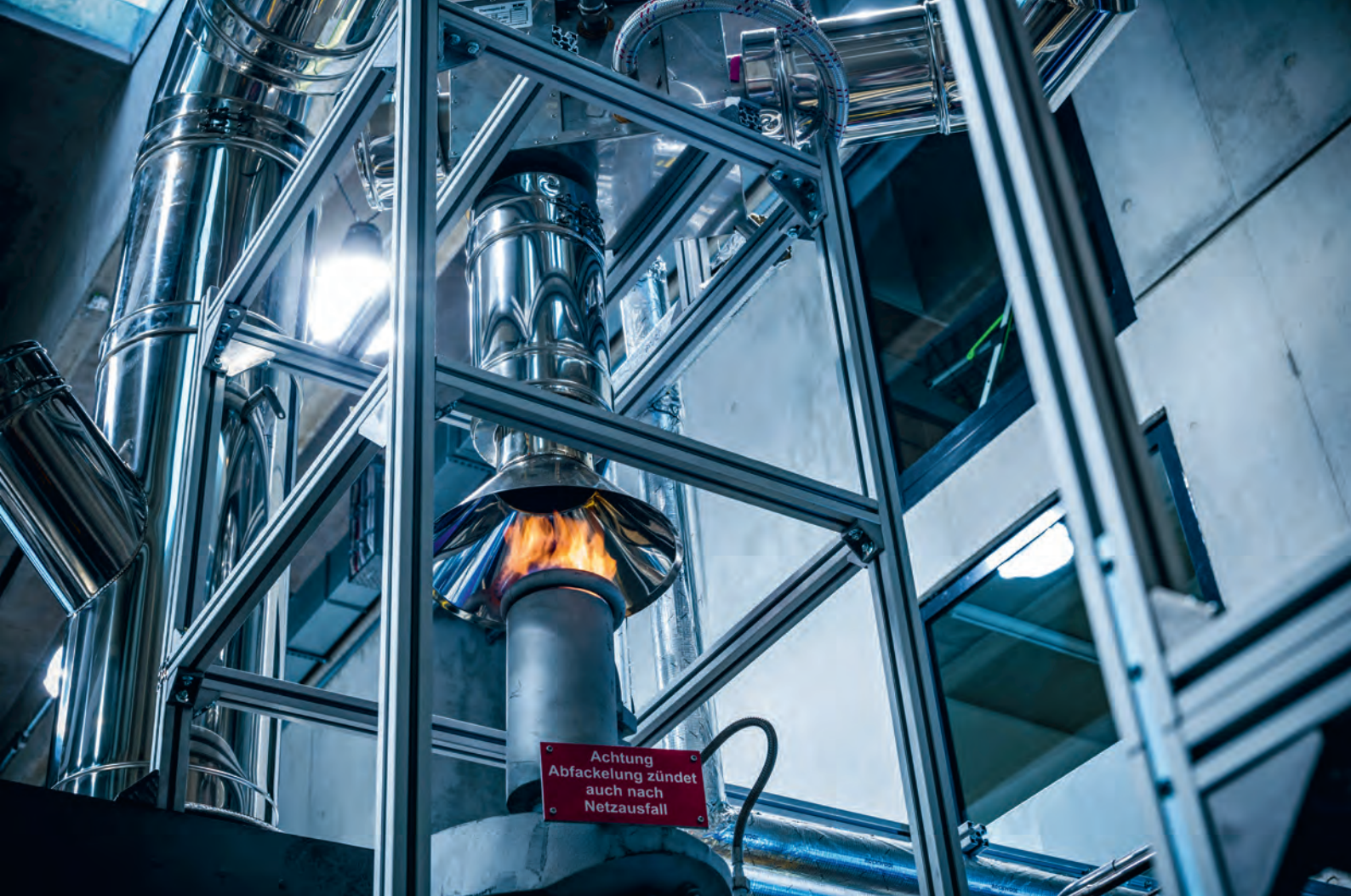
16 Surplus gas burner with waste heat exchanger
