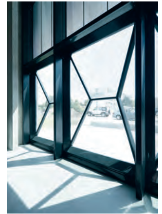
10 The south-facing element façade with light-directing lamellae in the gap between the insulating glass panes of the double glazing units (above) and the parametric façade elements (below)
